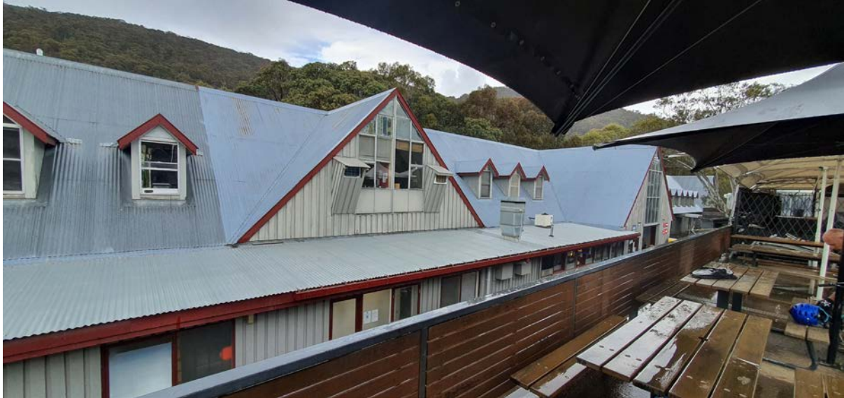
FIGURE 16 EXISTING ROOF CLADDING TO VALLEY TERMINAL BUILDING
