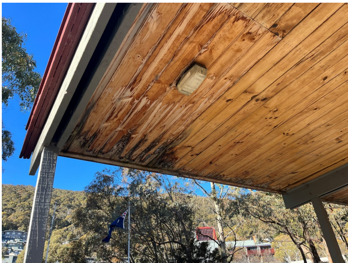
Ceiling Lining to be Replaced with Like-for-Like Material to Guest Services Building Awning.
