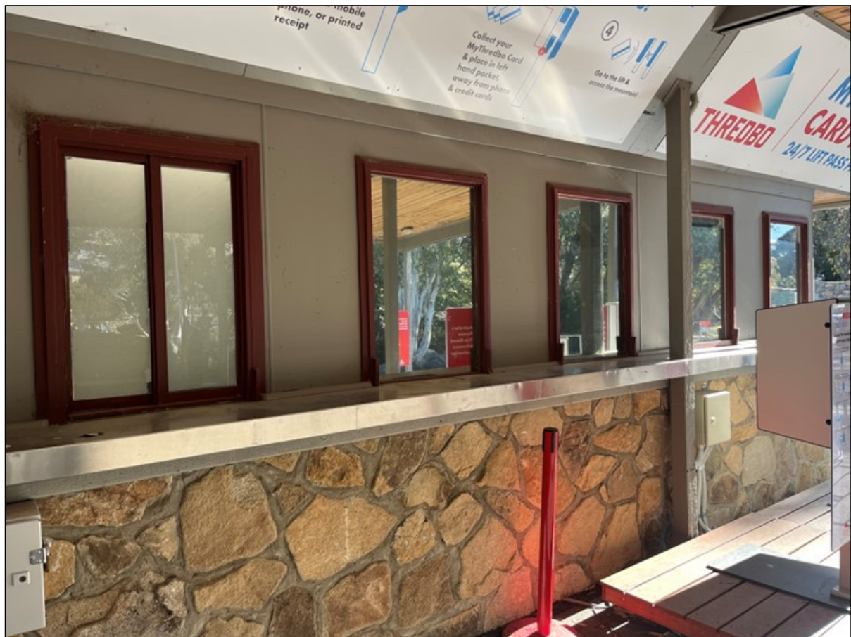
Ticket windows to be replaced within the existing timber frames.
